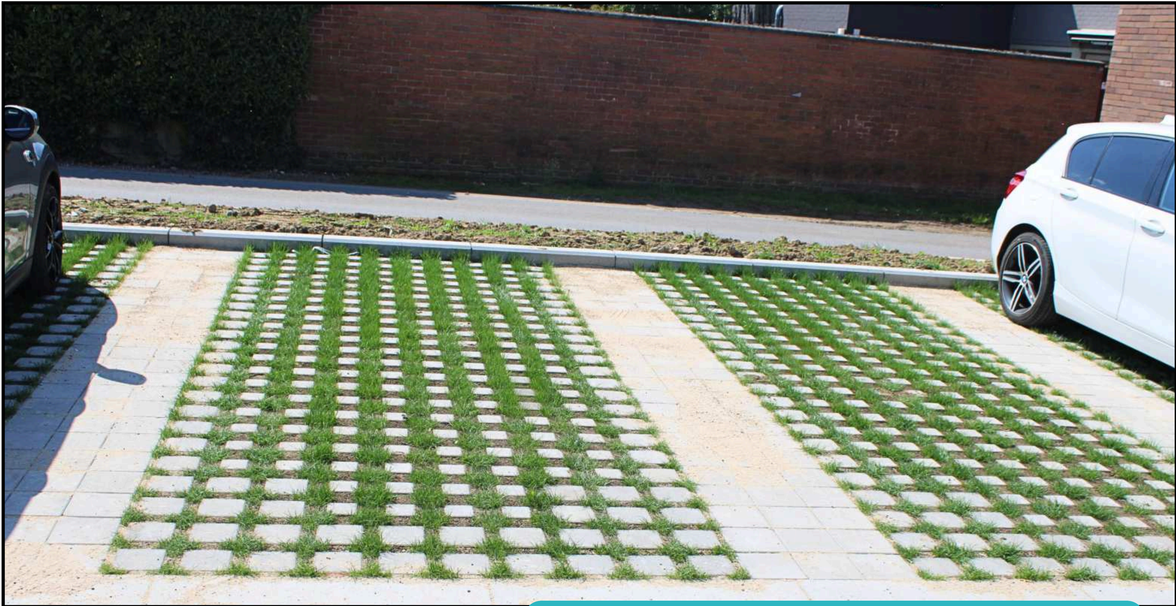
Project: Rusthuis Rekkem (fase 2)
